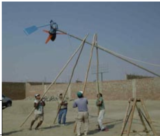
Photo 6 Raising a guyed tower with poles and ropes in Peru (Hugh Piggott)
